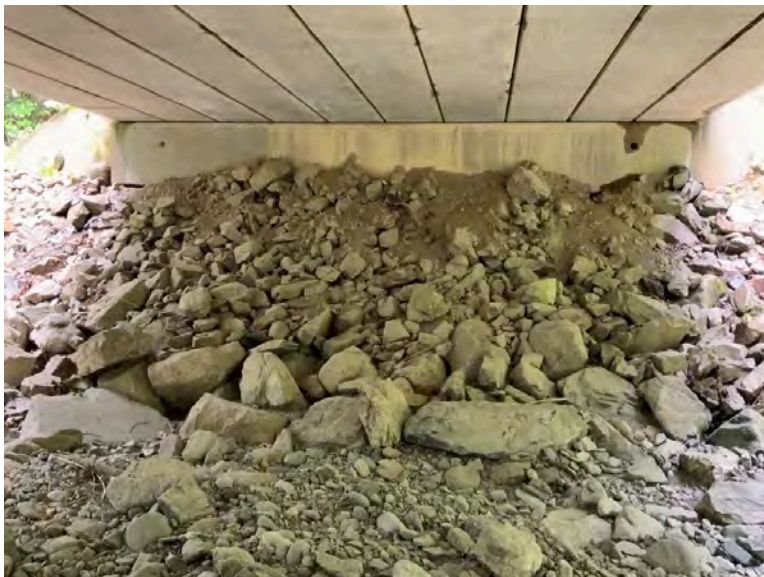
Right Bank Abutment when facing downstream
