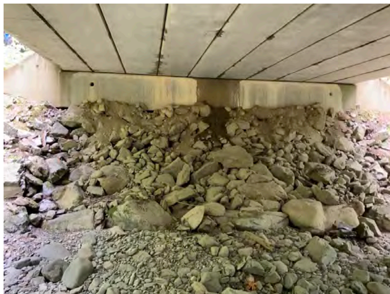
Left Bank Abutment when facing downstream
